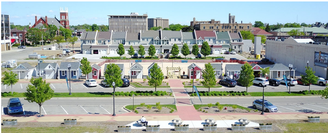
An aerial shot of the row of chalets at Western Market
