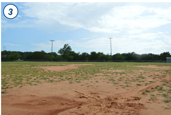
The baseball/softball field requires maintenance.
