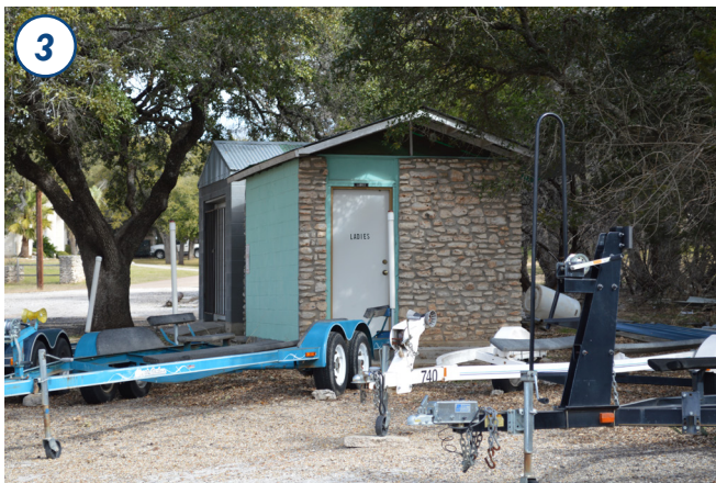
The existing restrooms on site do not appear to be open.
