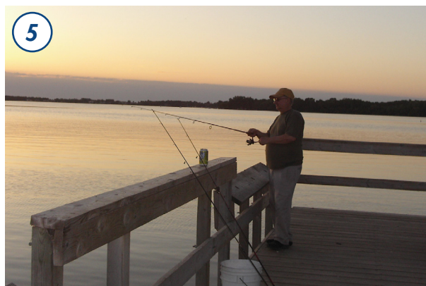
A cantilevered fishing pier provides a permanent fishing location without interfering with the lake.
