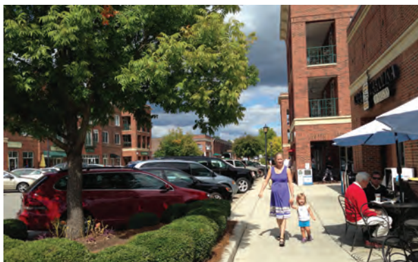
Meadowmont neighborhood in Chapel Hill, NC offers shops and businesses with residential upstairs.
