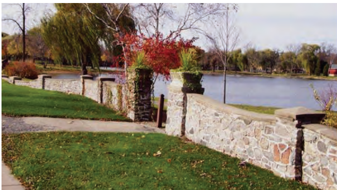
The glacial fieldstone wall at Riverside Park in Watertown, Wisconsin uses natural, local stone.
